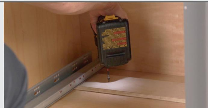
Secure the base unit by screwing through the 8 pre-drilled holes in the plywood runners with coarse-thread wood screws. #6 X 1" screws provided.
