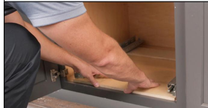
Place the base inside the cabinet. Center it left to right, ensuring proper clearance for hinge or door protrusion.
